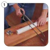
Cut PVC pipe to length with a hacksaw or a reciprocating saw equipped with a fine-toothed blade.
