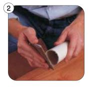
Smooth the rough-cut pipe ends, inside and out, with fine-grit sandpaper.
