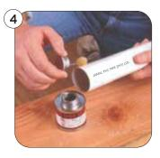
Immediately push the fitting onto the pipe end, twist it slightly, and hold the joint for about 30 seconds.
