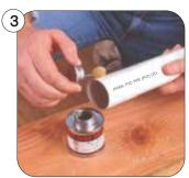
Apply a 1-inch-wide band of PVC cement around the end of the pipe only not to the fitting.
